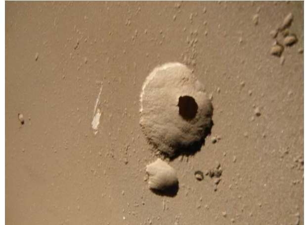
Figure 10 - MIC damage evident underneath tubercle. Image was taken after abrasive cleaning
