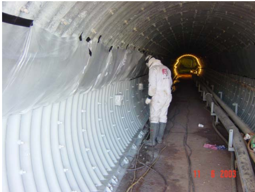
Fig X: Photograph showing spray application of “splash zone” coating to tunnel wall.
