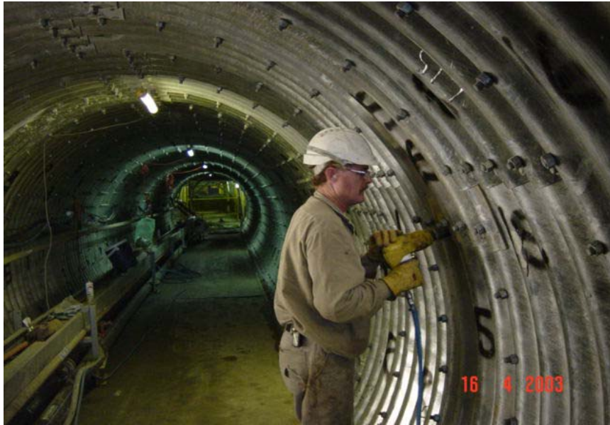
Fig VIII: Photograph showing new tunnel sections being torqued after installation.
