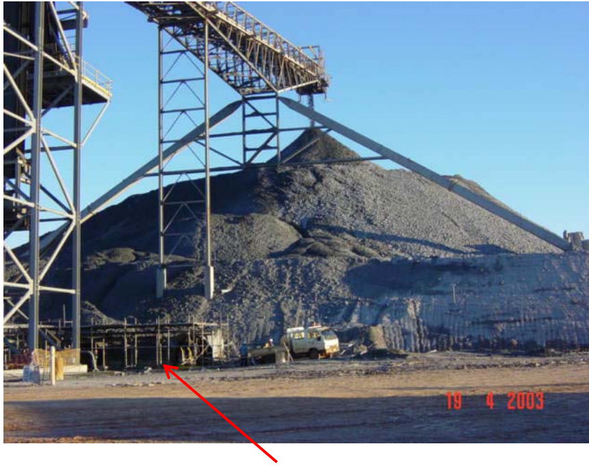
Fig I: General view of main ore stockpile. Note Emergency Escape Tunnels at base of stockpile.
