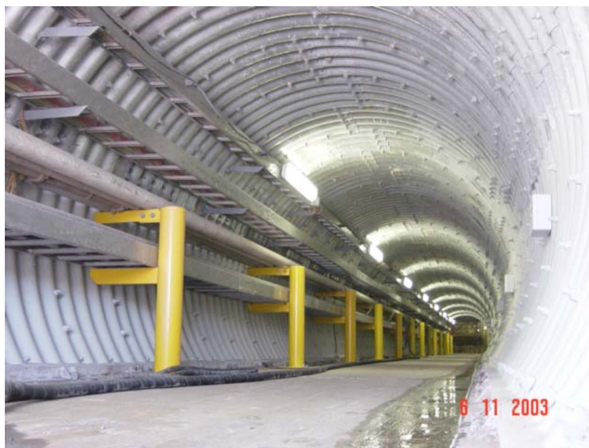
Fig XIII: General view of refurbished tunnel with all service relocated.
