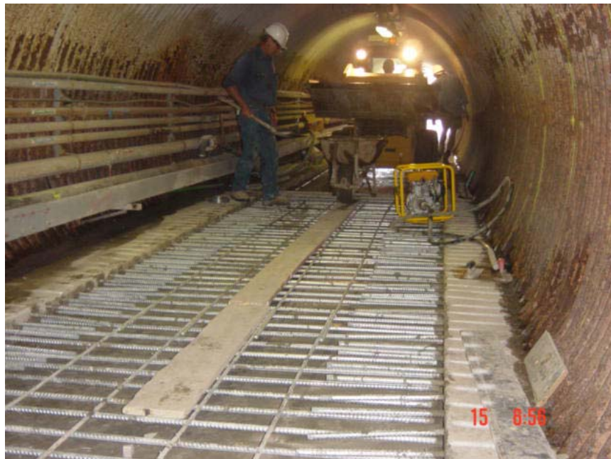
Fig VI: Photograph showing existing concrete floor strengthening prior to undertaking tunnel placement.
