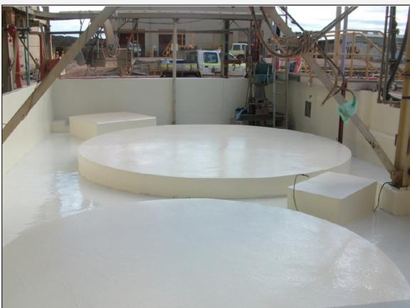
**Protective coatings** are another method of reducing negative effects on concrete. Recommendations of suitable coatings for the long term protection of concrete against these chemicals, and other causes of damage, such as impact and abrasion, can be undertaken by Extrin. Specifications for the correct preparation and application of recommended coating products is also part of our expertise.
